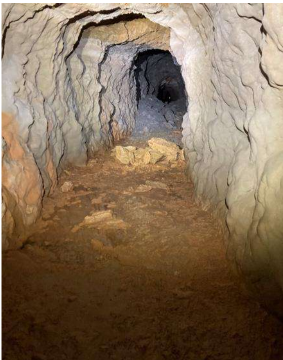
Figure 12 Éboulement PM 1500
