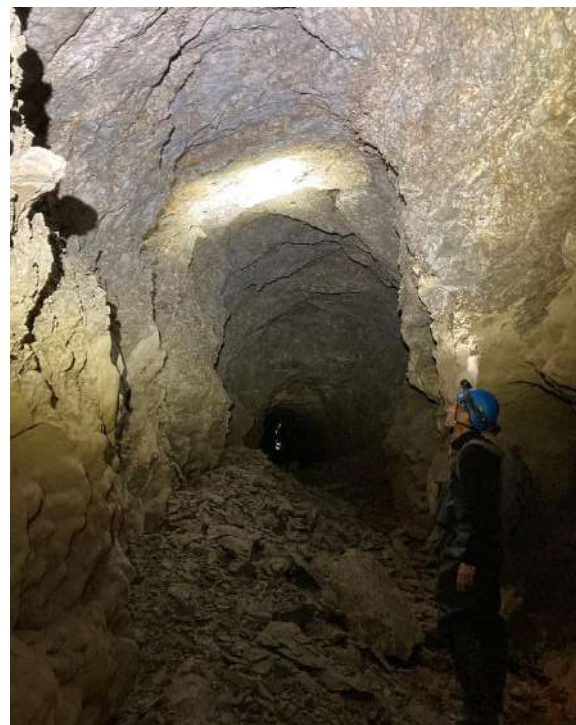
Figure 13 Éboulement PM 1500
