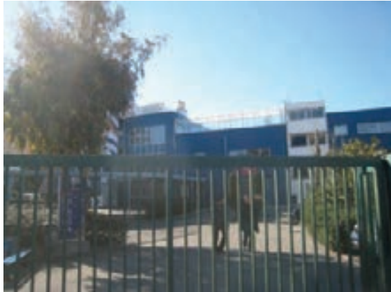
Figure 6 : Photo Institut de Formation Automobile (Source: Egis France)
