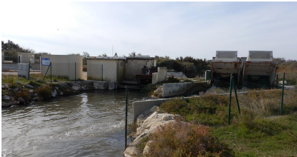
Figure 16 : Station de l'Eolienne (BRL i, 2015)
