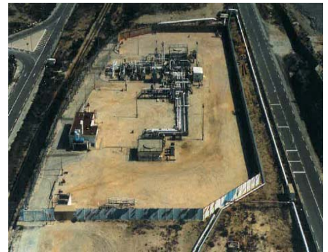
Géogaz – installations de surface
