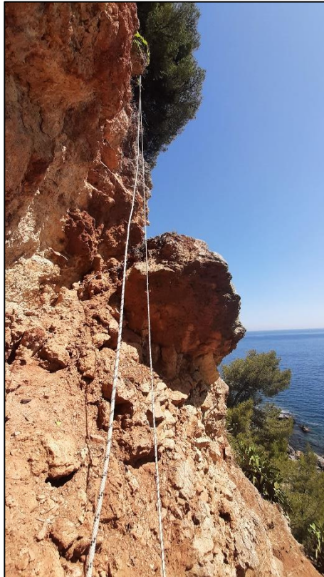
Figure 42 : Photo de M2
