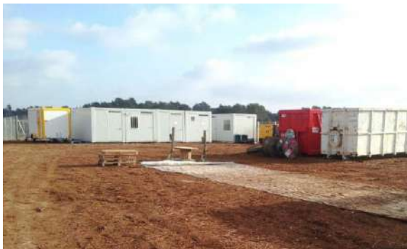
Installation de la base vie
