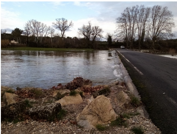
Illustration 23: Pont submersible de Villetelle -26-01-2020 15h-Source SPC GD
