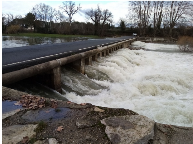
Illustration 22: Pont submersible de Villetelle -26-01-2020 15h-Source SPC GD
