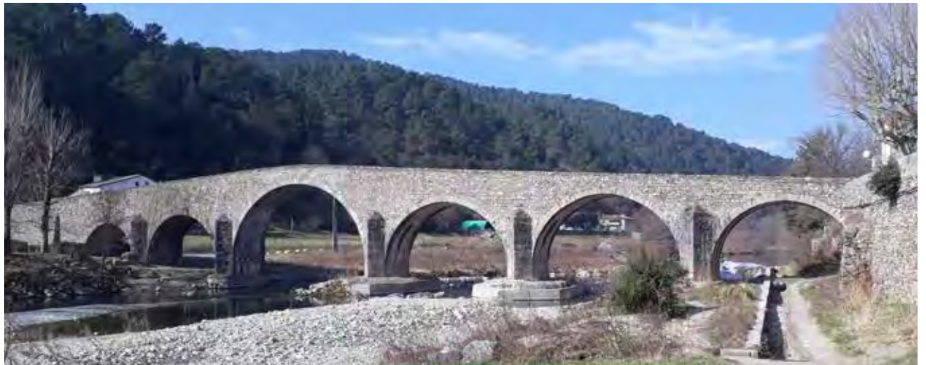
The St Jean du Gard bridge destroyed by the Gardon River and view of the bridge today, which contains lighter coloured stone dating back to repairs to its highest arch.
