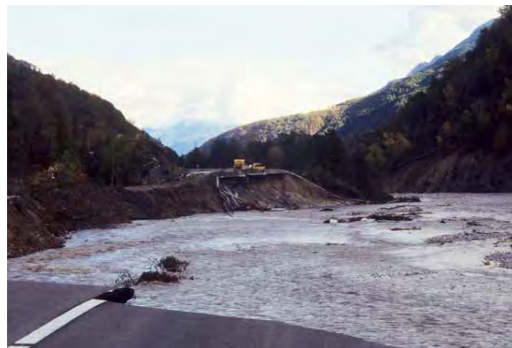
Transport infrastructure was severely affected throughout the river catchment*, such as here at Puget-Théniers (06) where the road and railway line were washed away.
