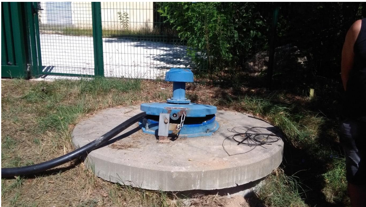
Figure 22: Photo du captage F3 Du champ captant de Vidauban (ICEA, 02/09/2016)
