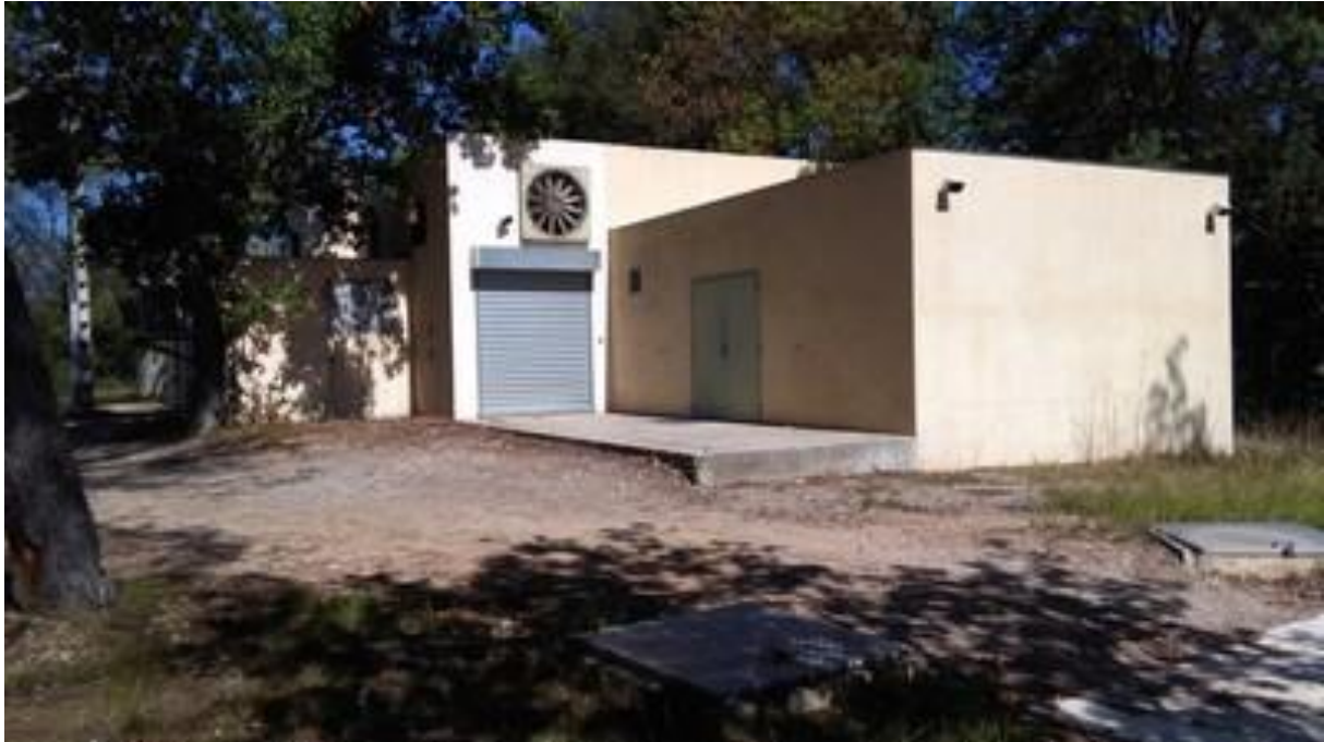
Figure 8 : infrastructures du SIAE (ICEA 02/09/2016)
