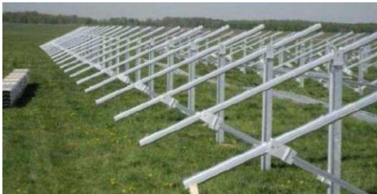
Exemple de structures de support sans modules (Source : VOLTALIA)
