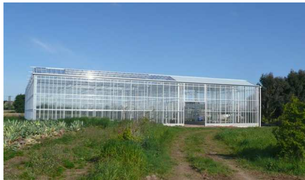
Serres Cressonnières Boé 1,2 hectare – 1 MWc installé
